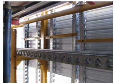
Above: Steel framing provides a solid and secure work platform.
