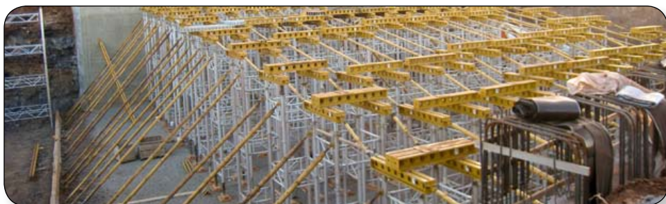
Bridge deck shoring with EFCO E-Z DECK and SUPER STUDs
