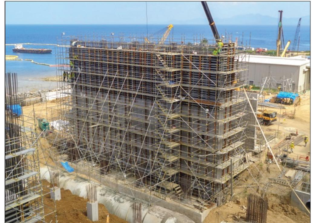
*EFCO designed 98'-6" (30 m) long x 20' (6 m) high E-BEAM® and SUPER STUD® wall gangs to easily construct the structure in three lifts.*
