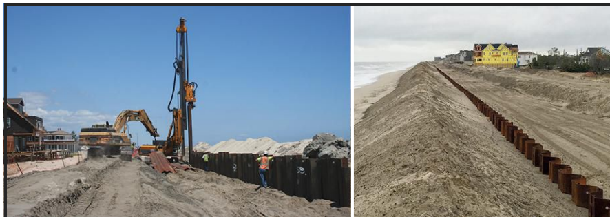
Wide flange beams are driven to depth for a redesigned king pile wall.
