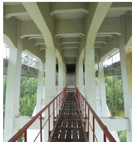
BrandSafeway engineered a custom anchoring system for the suspended access system used on the renovation of the Caracău Viaduct railway bridge in Romania.
