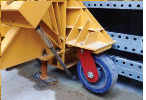
Gangs can be rolled around between pours on four swivel wheels.
