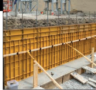
Foundation Wall, Ames, Iowa
