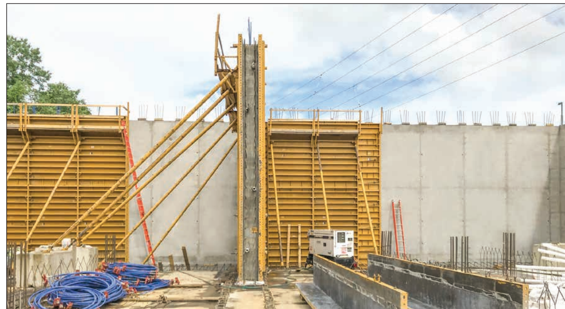
The EFCO PLATE GIRDER ® system was the perfect formwork for the 24' (7.3 m) to 29' (8.8 m) tall walls and columns.
