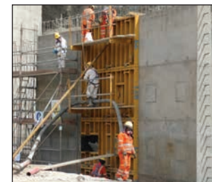
UNACEM Cement Clinker Plant, Tarma City, Peru
