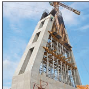
Bridge Over Ariari River, Puerto Llerasm, Colombia
