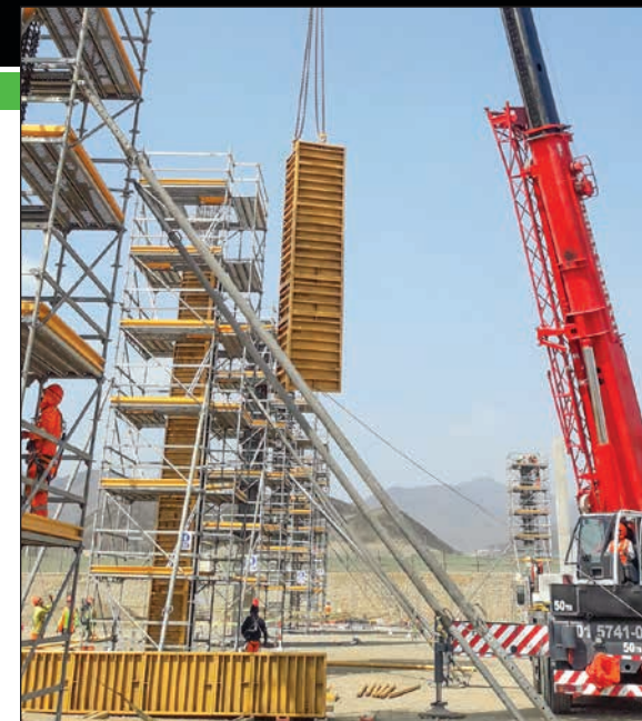
Six sets of EFCO LITE® forms were used to complete six columns a day.
