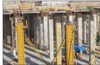
Underground Storage Basin, Louisville, Kentucky
