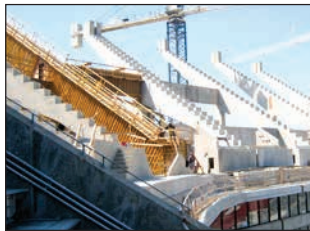
Crimson Tide Stadium Expansion, Tuscaloosa, Alabama
