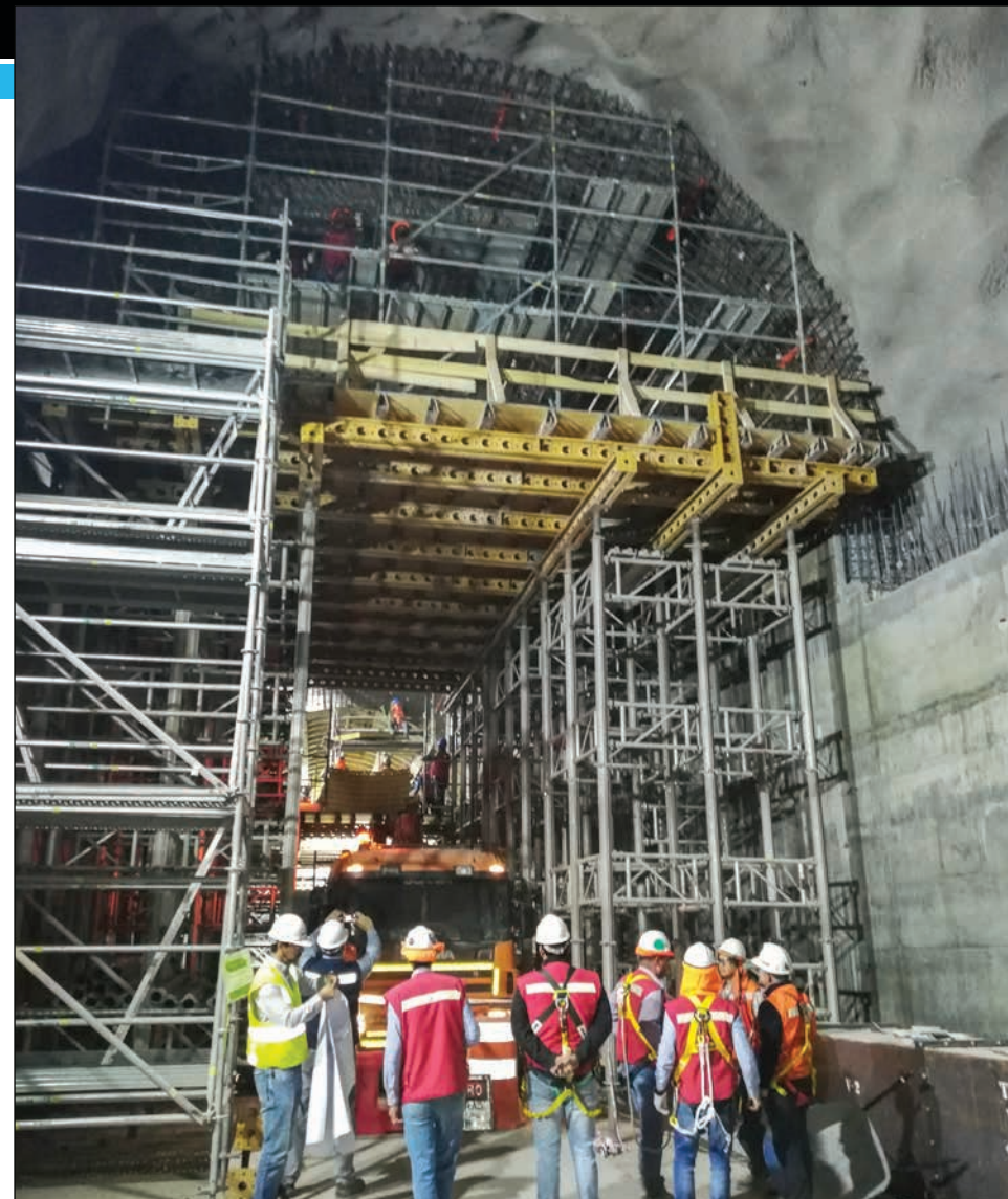
E-Z DECK® towers supported work platforms and were positioned to provide enough space for work vehicle traffic to continue through the tunnel.
