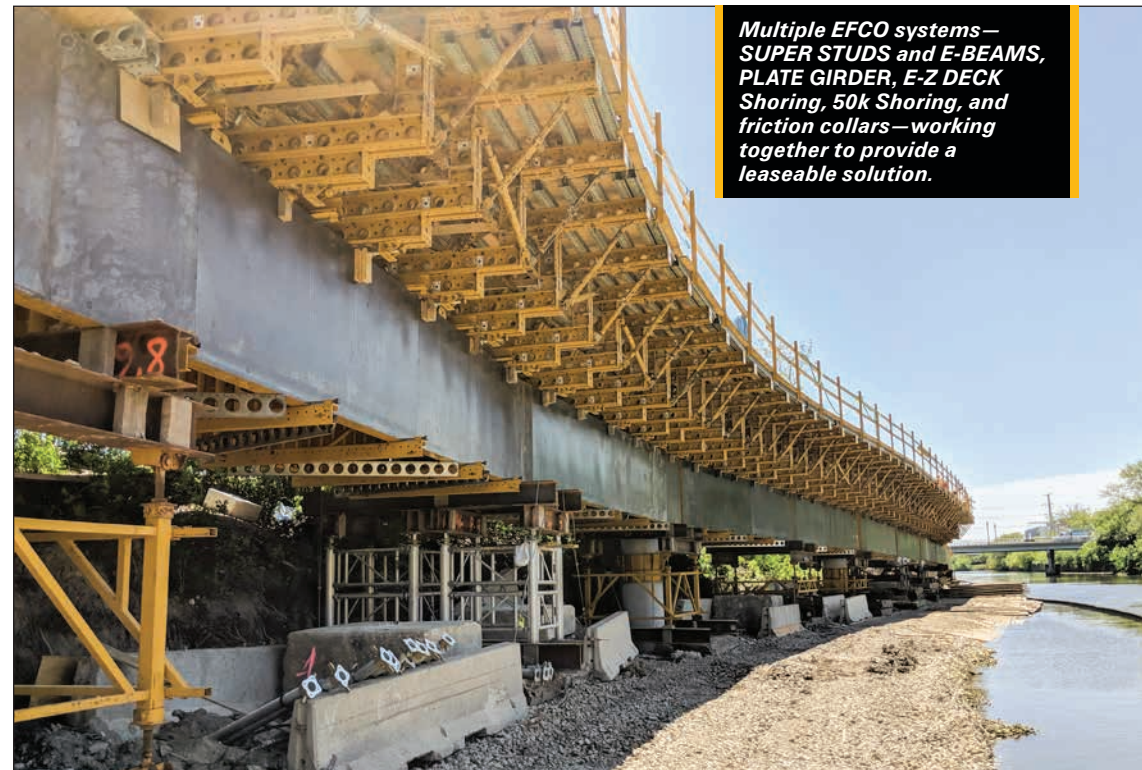
EFCO was able to build custom-shaped tubs out of SUPER STUDS® and E-BEAMS® that could be adjusted to handle the curve, camber and bank of the bridge.
