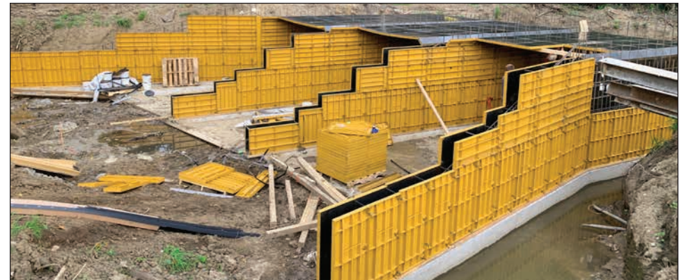
Box Culvert, Columbus Junction, Iowa
