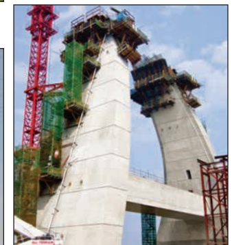
Dapeng Pylon Bridge, Pingdong, Taiwan
