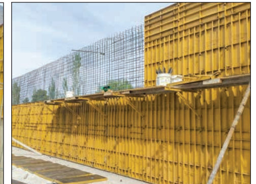
Cinco Saltos Water Treatment Plant, Cinco Saltos, Neuquen, Argentina
