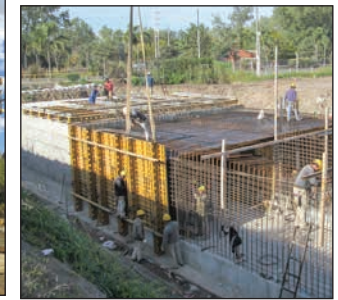
Box Culvert, Canning, Argentina
