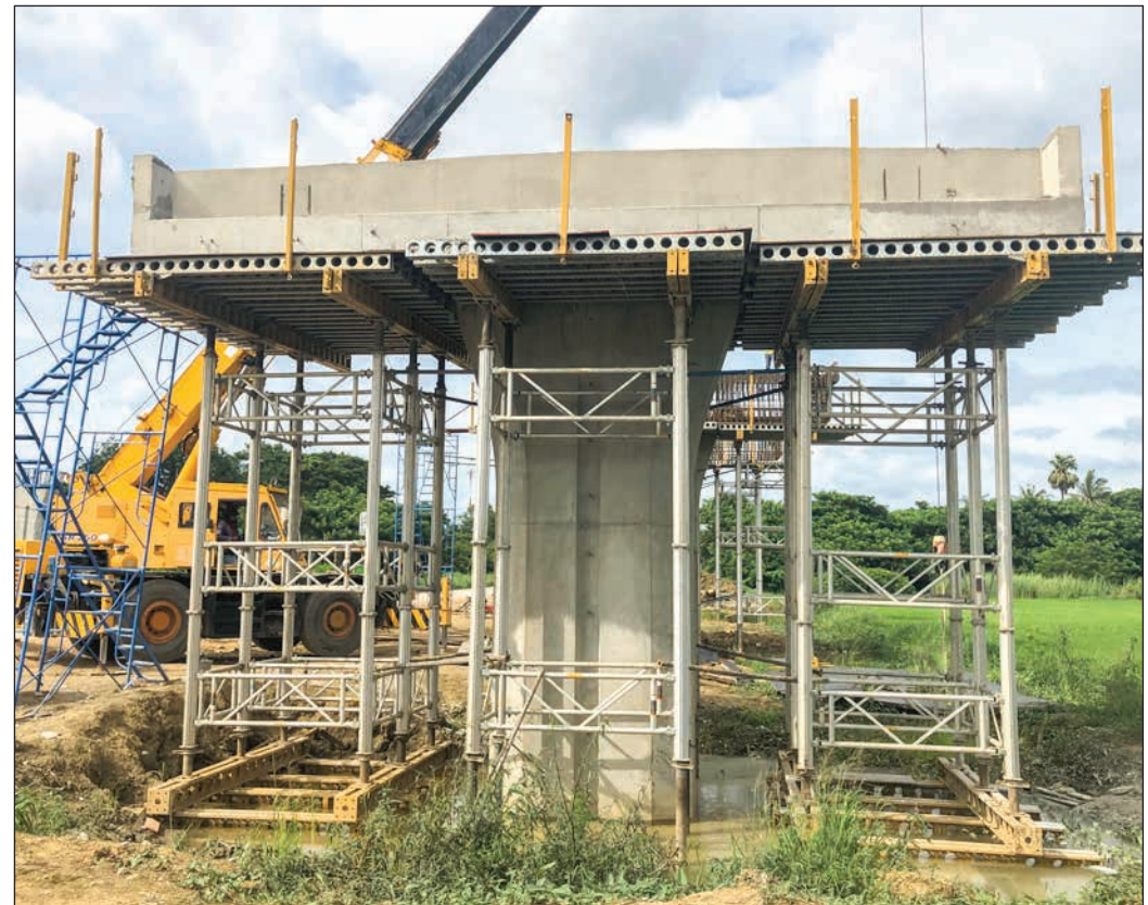
EFCO SUPER STUDS® were used below the E-Z DECK® shoring system. This allowed work to continue during the rainy season in Thailand without any concerns of not working on solid ground.
