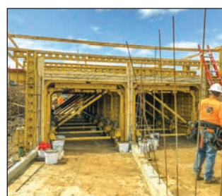
Box Culvert, Kihei, Maui, Hawaii
