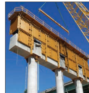
Bridge Over the Missouri River, St. Louis, Missouri
