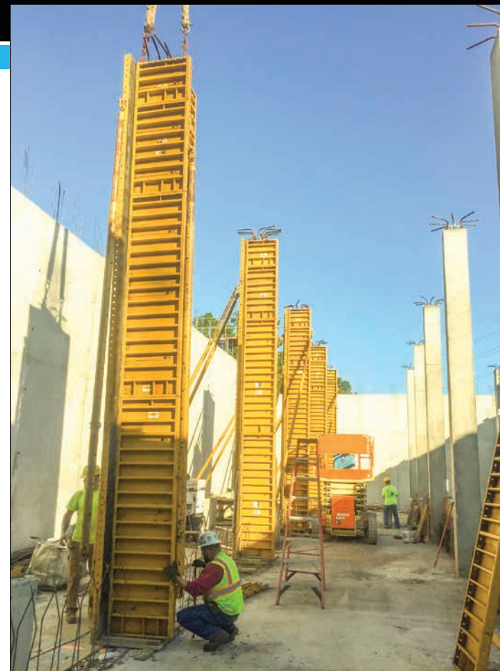
The EFCO PLATE GIRDER ® system was the perfect formwork for the 24' (7.3 m) to 29' (8.8 m) tall walls and columns.
