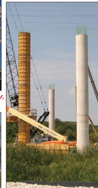
Murray Baker Bridge, Peoria, Illinois
