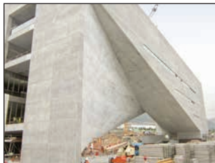
Roberto Garza Sada Center, Monterrey, Mexico
