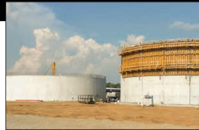
Digester Tanks, Rosendale, Wisconsin
