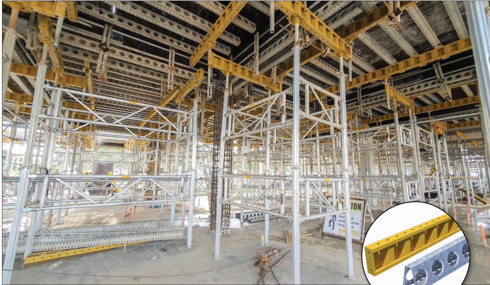
The combined strength of the PRO 4 ® Post and the Z-BEAM ® stringer and E-BEAM ® joist means using fewer posts.
