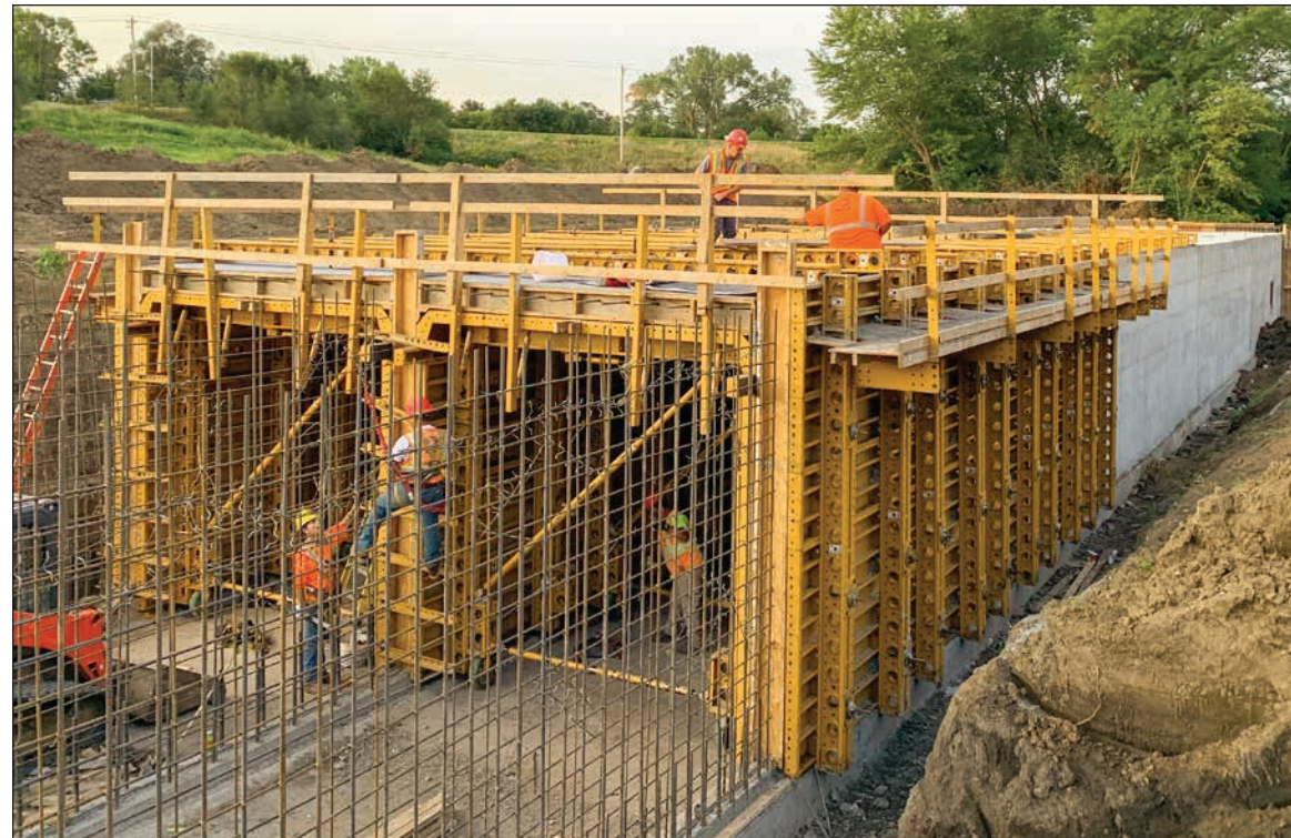
The Traveler was constructed with EFCO's standard EFCO LITE® wall system along with the needed box culvert system accessories.
