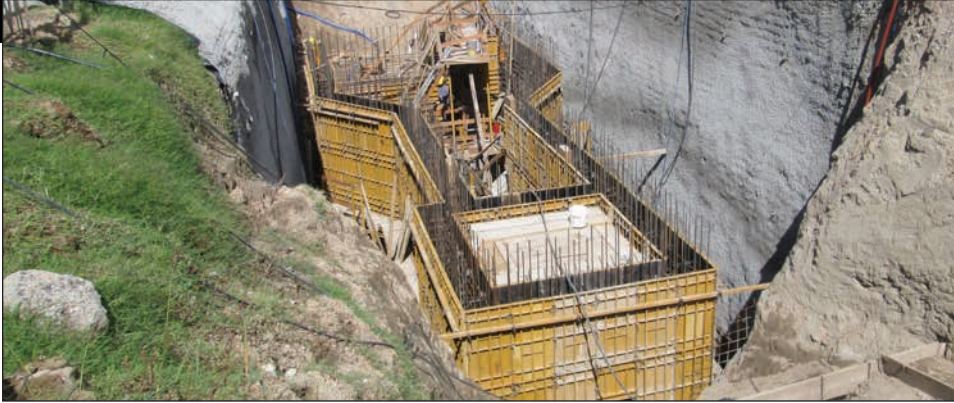
Pump Station Benavidez, Buenos Aires, Argentina
