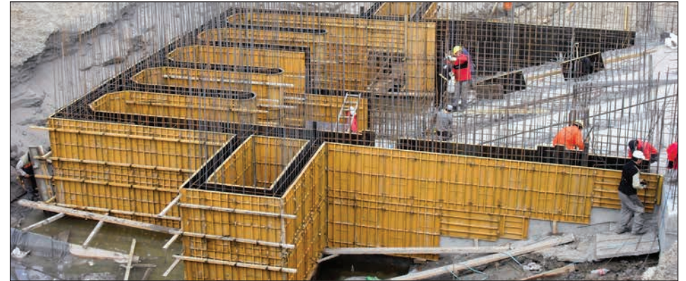
Cerro Viento Bridge, Panama City, Panama
