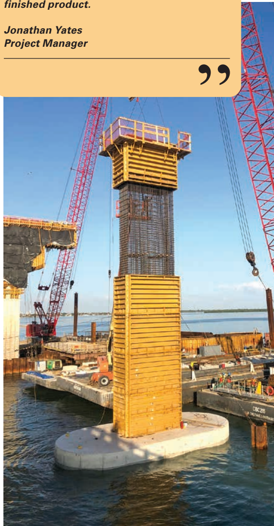
For the columns, AB chose the EFCO tieless PLATE GIRDER column forms.
