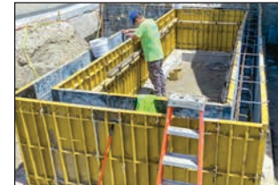
Waste Water Treatment Plant, Ames, Iowa
