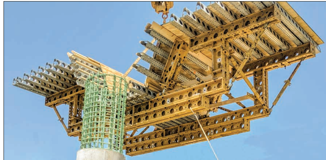
EFCO was able to build custom-shaped tubs out of SUPER STUDS® and E-BEAMS® that could be adjusted to handle the curve, camber and bank of the bridge.
