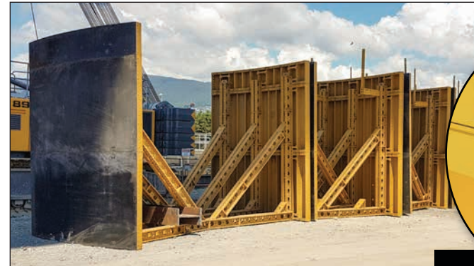
EFCO REDI-RADIUS® formwork was bolted to SUPER STUD® bracing and staged ahead of being placed with the crane.
