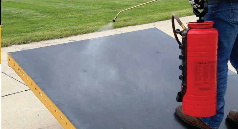
Begin spraying at the top of the form and apply a very thin and even coat.
