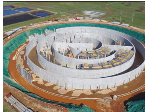
Blackman Water Treatment Plant, Springfield, Missouri
