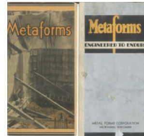
W. A. Jennings sold formwork for Metaforms before starting Economy Forms.
