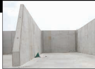
Manufacturing Facility, Mount Pleasant, Tennessee
