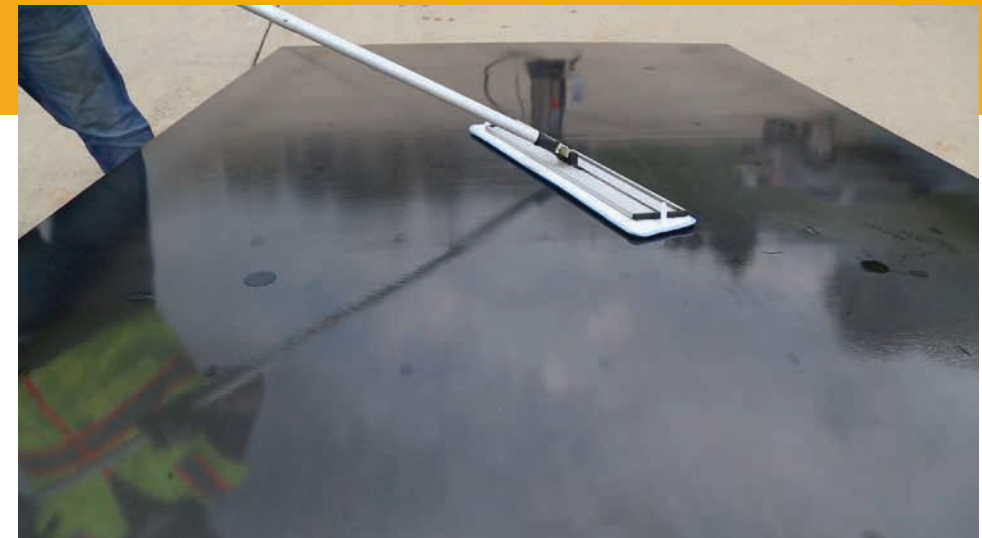
For best results, after applying the release agent, use a microfiber mop to ensure a nice even coating. This will also help eliminate drips and runs.
