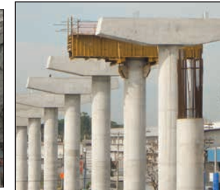
Line 2 of the Panama Metro, Panama City, Panama
