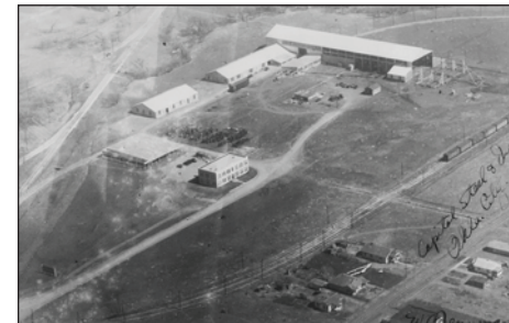
One of W. A. Jennings’ early jobs as a civil engineer was at Capitol Steel & Iron in Oklahoma City
