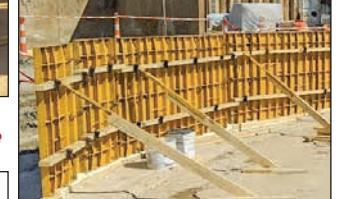
Northeast Boundary Tunnel Washington, D.C.
