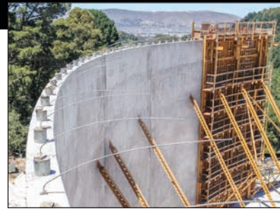
Harry Tracy Water Treatment Plant, San Bruno, California
