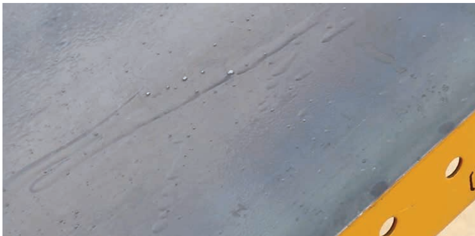
Apply the release agent as thin as possible while still being able to achieve complete coverage. Application of release agent has been applied too thick in the picture shown above. Make sure there are no visible runs or drips on the surface during or after application.
