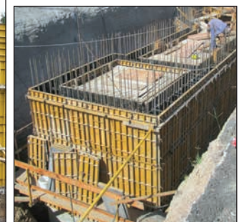
Pump Station Benavidez, Buenos Aires, Argentina
