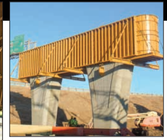
Red Highway Improvement Project, Wichita, Kansas
