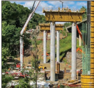
I-91 Bridge Replacement Windsor, Vermont
