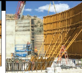
Water Treatment Facility, Brewster, Washington
