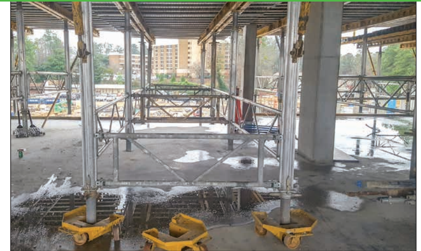
Crazy Wheel Dollies attach to the bottom of the E-Z FLYER tables so they can be moved without tear-down and reassembly.
