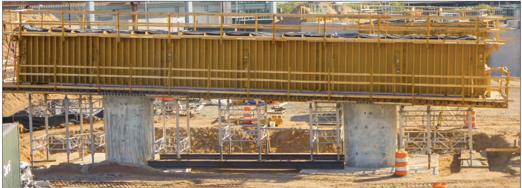
EFCO's PLATE GIRDER® system provided a smooth, architectural finish.
