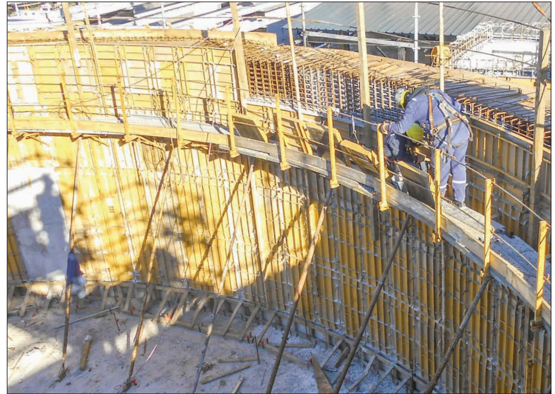
Standard HAND-E-FORM ® panels when used with HAND-E-FORM flexible panels will form tanks and curved walls.
