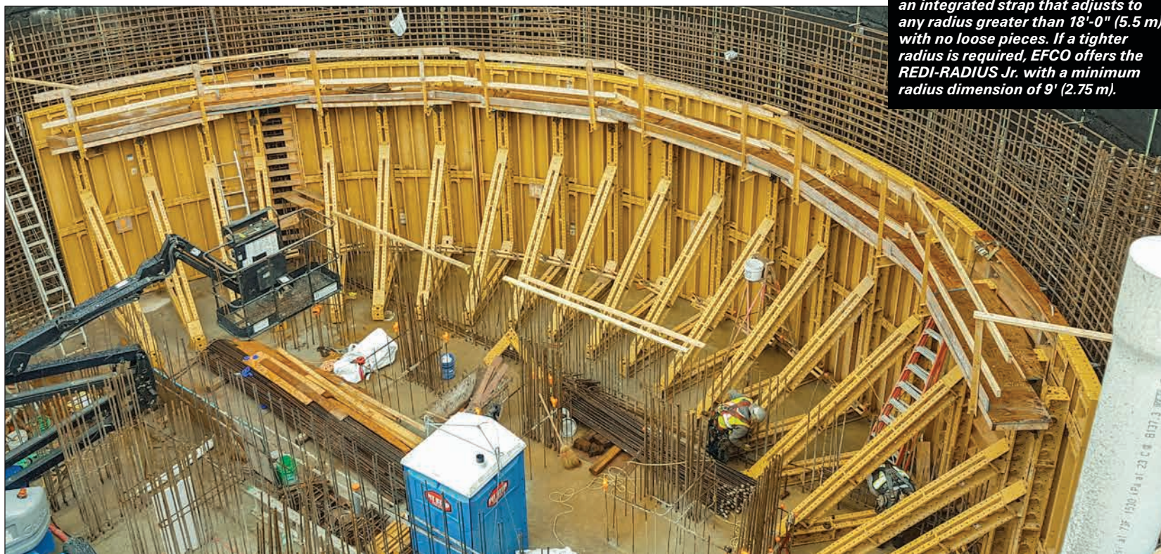
EFCO REDI-RADIUS® formwork was bolted to SUPER STUD® bracing and staged ahead of being placed with the crane.
