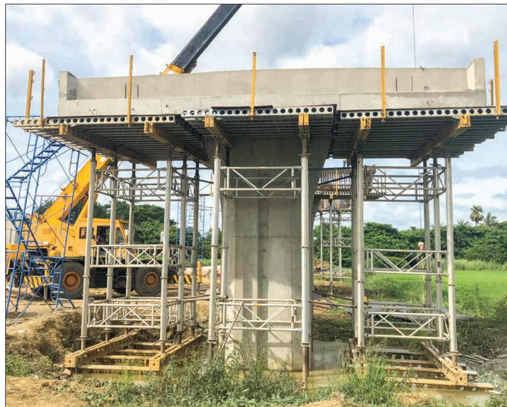
EFCO SUPER STUDS® were used below the E-Z DECK® shoring system. This allowed work to continue during the rainy season in Thailand without any concerns of not working on solid ground.
