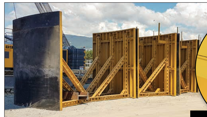
EFCO REDI-RADIUS® formwork was bolted to SUPER STUD® bracing and staged ahead of being placed with the crane.
