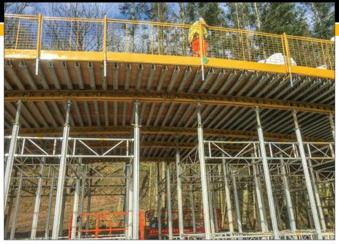
EFCO E-Z DECK® shore towers support the arched bridged during erection.
