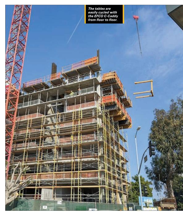
EFCO provided PLATE GIRDER® beams extending roughly 9' (2.7 m) from the building footprint below to support the E-Z DECK® tables below cantilevered cast-in-place deck pours.
