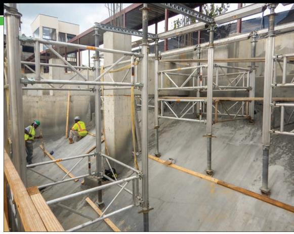
For the slopping base, EFCO's solution was to attach the EFCO Swivel Head Adapter on the bottom of the E-Z DECK® posts to stabilize the shore towers and support the 12" deck slab.
