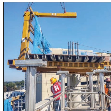
Cycling the perimeter beam towers with EFCO's new 3.5K (15.6 kN) adjustable C-Caddy.
