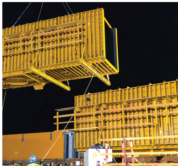
Large gang crane handling without the need for stiffbacks.
