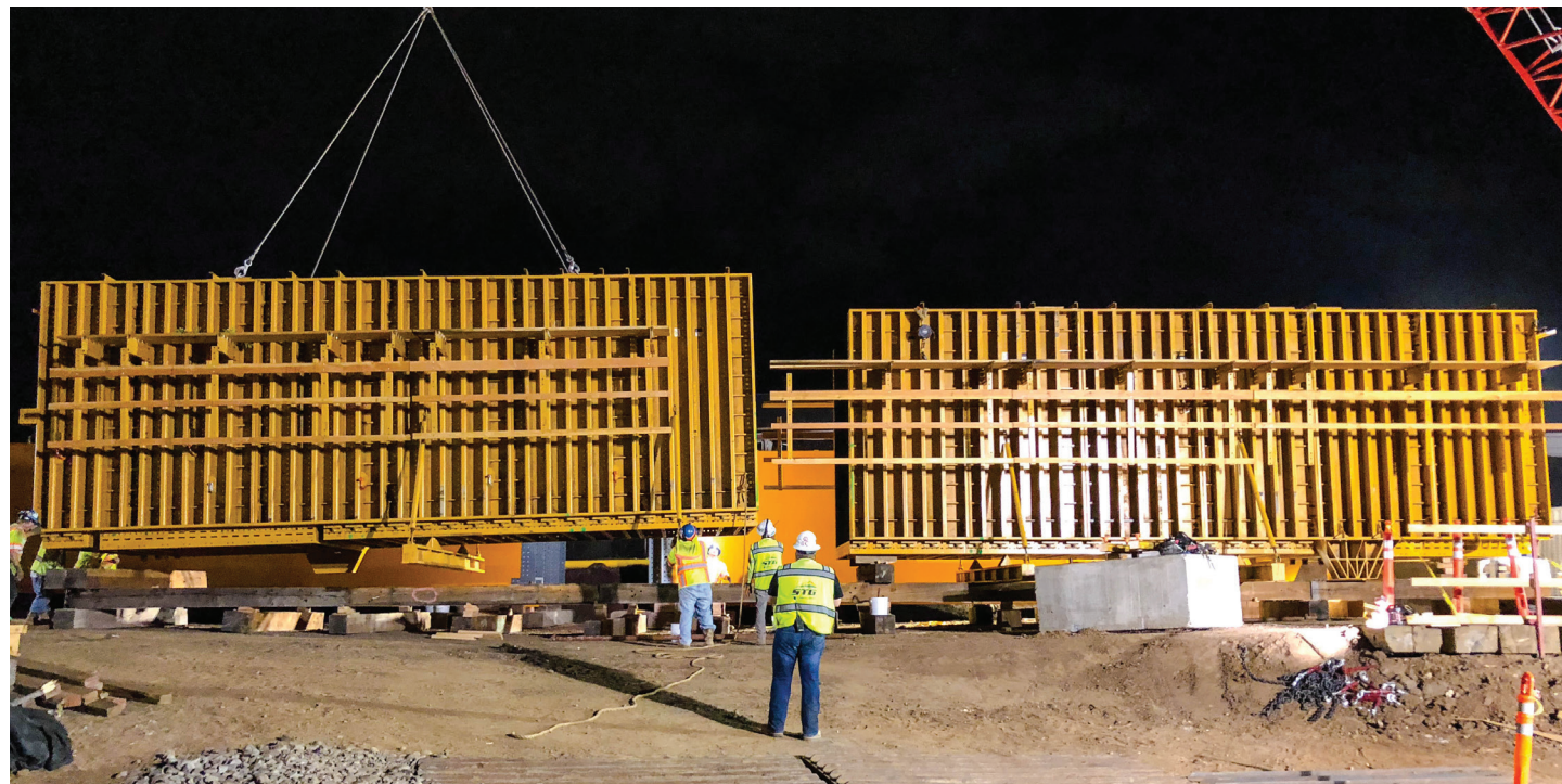
EFCO SUPER PLATE GIRDER has over twice the moment carrying capacity of classic PLATE GIRDER to form larger, longer spans without shoring to the ground.
